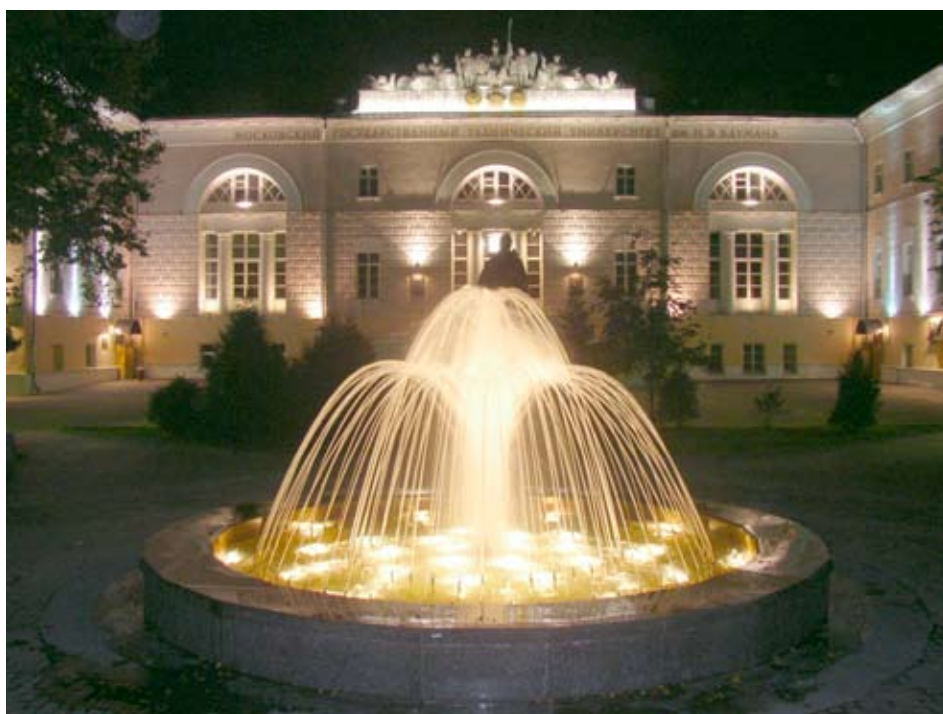
Inner courtyard of the Moscow State Technical University; the demonstration and training centre with CNC machining systems of vhf is situated in the building
